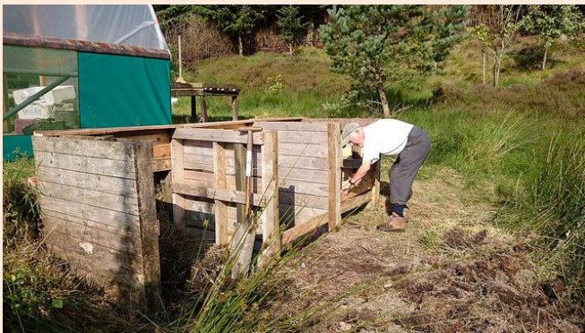
Building composting bins at Glenlude
