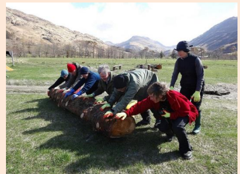
Building benching on Long Beach campsite
