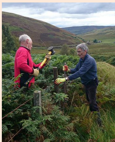
Repairing fences at Glenlude
