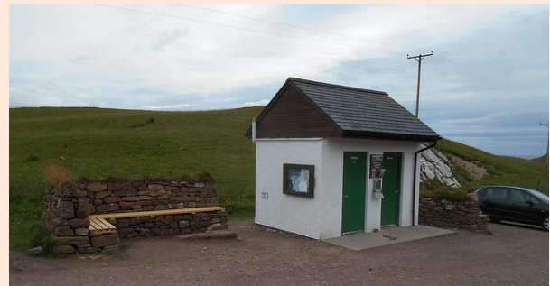
Repainted toilet and new woodwork at Sandwood car park
