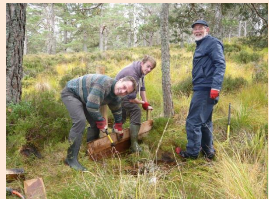
NE Members group ditch blocking
