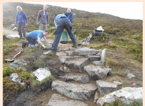
New stone pitching constructed on Schiehallion path
