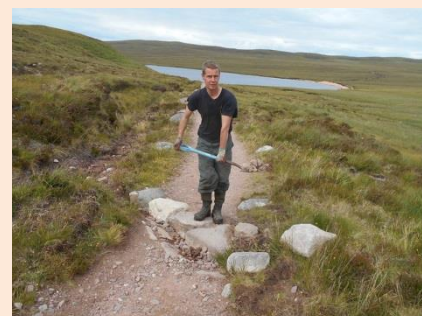
Path maintenance at Sandwood
